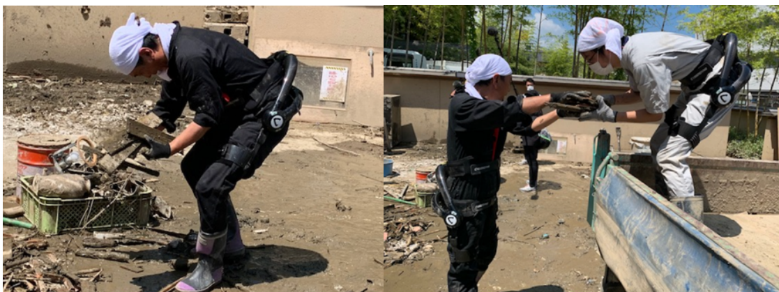
July 30, 2020 (disaster recovering activity in Hitoyoshi, Kumamoto Prefecture)
